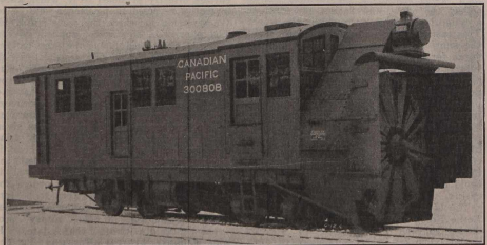
Fig. 4.—1911 Type of C.P.R. Snow Plow with Cut Wideners.
