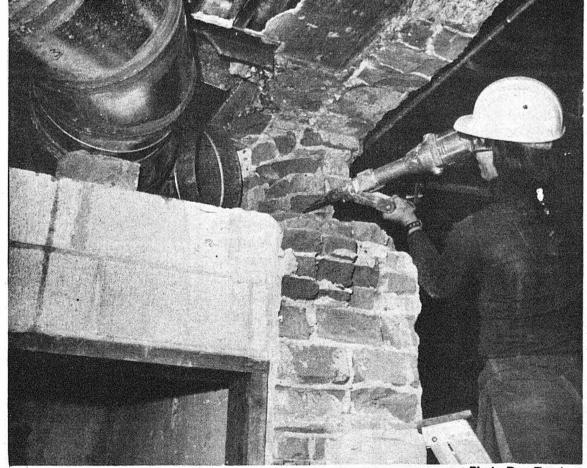
Athabasca Hall gets \$1.8 million facelift. Jackhammers jolt the foundations of Athabasca Hall, making room for upgraded ventilation. The entire interior of the building is being demolished, leaving only the outer shell of one of the oldest buildings on
