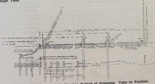
Fig. 3.—Longitudinal Section Showing Method of Dropping Tube in Position.
