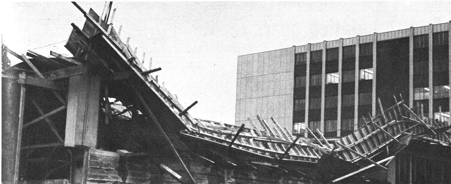
**NERVOUS BREAKDOWN**—Faced with the prospect of 30,000 students, a section of the new parkade collapsed under the strain Thursday. The collapse spewed semi-hardened cement over the site. For lack of a more concrete suggestion, why not leave it as it is and label it "Progress?" This campus needs a little culture, and besides students are last on the parkade's occupancy list, anyway.
