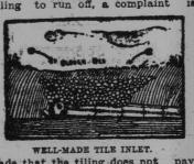
age. Where soil is of a mucky nature, the illustration shows a good plan of filling in around the inlet. This plan, however, is not necessary eight inches of the surface, so the plow will not strike the stone. This will let the water off freely, yet keep soil in good shape. A large
