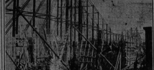
Work in Connection With The New Bridge at the Reversing Falls by The Standard's Staff Photographer.
