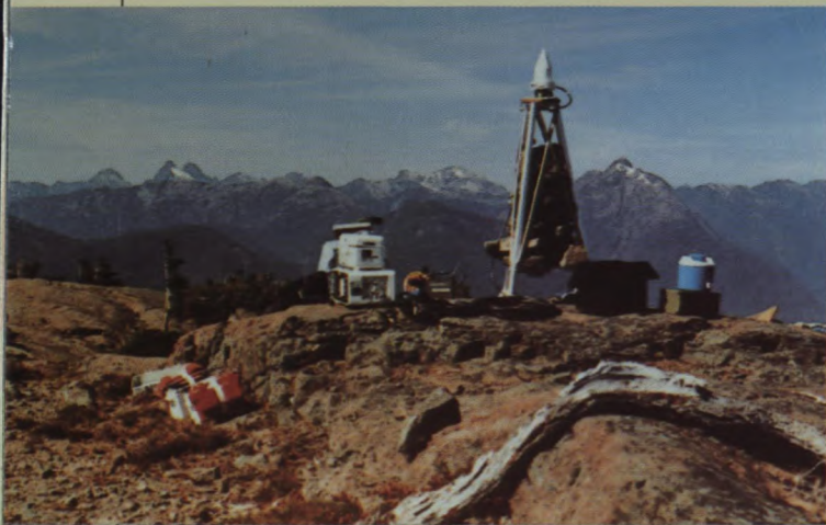
A satellite Global Positioning System (GPS) site and receiving antenna centred over a geodetic marker.
