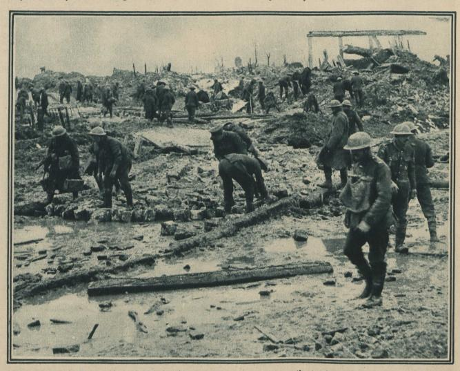
Before the light railways can be laid it is of course necessary to prepare the tracks, and this wherever possible is done along a road. Here Canadian Pioneers are endeavouring to re-make a road which has been battered to bits by shell fire. It is at times almost impossible to say where the road originally ran.
