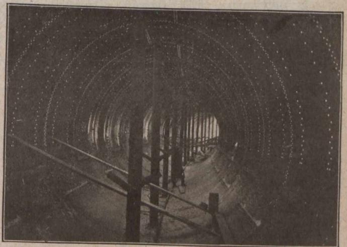
FIG. 2—DOUBLE-RIVETED LAP JOINT IN 18-FT. DIAMETER PIPE, ONTARIO POWER CO.
