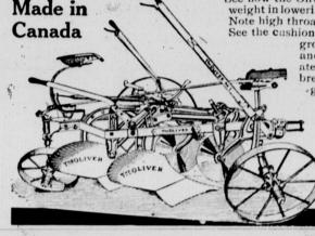
See how the Oliver foot lever is placed so that the operator can use his entire weight in lowering bottoms, easily penetrating hard ground or heavy vegetation. Note high throat and wide clearance between bottoms which prevents choking. See the cushion spring on land wheel which insures a level furrow on uneven
