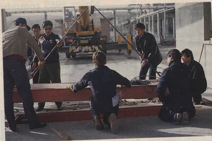
Technicians from Canadian Scale Company Limited in Toronto install a fully electronic in-motion truck scale system in a coal handling facility in Taiyuan, Shanxi, People's Republic of China. It is the first of its type to be installed in the country.
