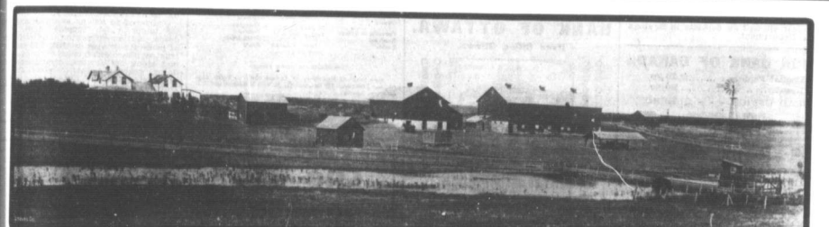
Western Farm Homes—Buildings of G. and B. Spring-Rice, Pense, Assa.
