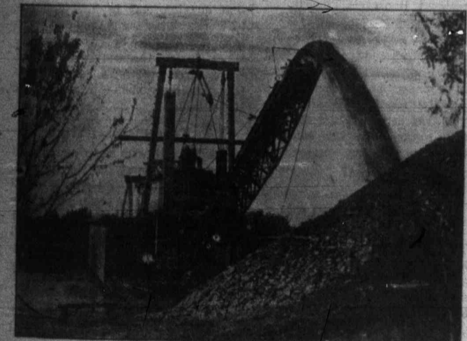
Steam Dredge Operating in Connection With a Conveyor.
