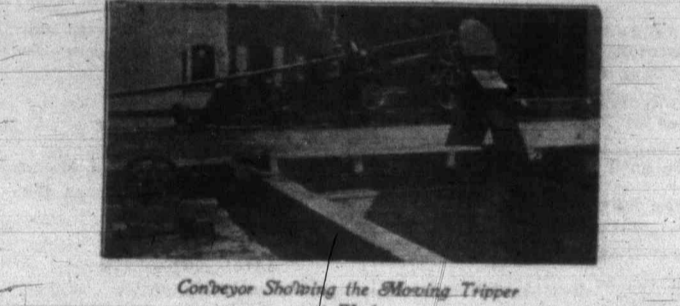
Conveyor Showing the Moving Tripper at Work.
