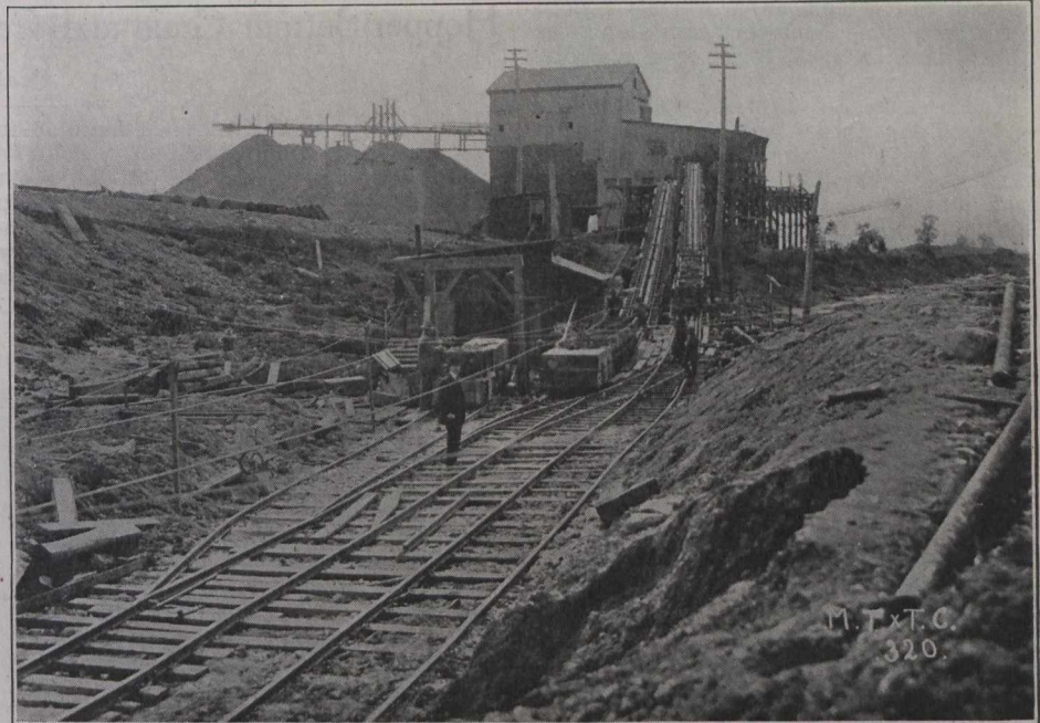
Mount Royal Tunnel—West Portal, Crushing Plant and Tipple.
