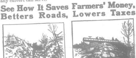
This picture is from a photo of a washout fourteen feet deep in the Township of Darlington, caused by use of cement tile for drainage purposes. The township authorities have replaced that with Pedlar Perfect Culvert, forty feet in length by three feet in diameter; strongest, easiest laid and most durable they could get.
