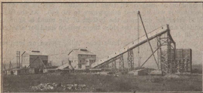
CRUSHER PLANT—PRIMARY TRAYLOR CRUSHER AT LEFT, GYRATORIES IN CENTRE, SCREENS ABOUT TO BE ERECTED AT RIGHT—CAPACITY, 3,500 CU. YDS. DAILY
