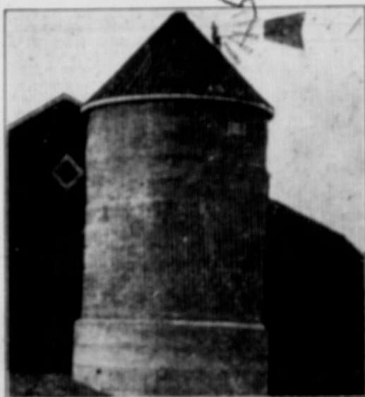
Stave silo on farm, Turner's farm, Carroll, Man. Stave silos are solid and durable but freeze rather badly. This one is partly underground, making that part like a 'pit' silo.
