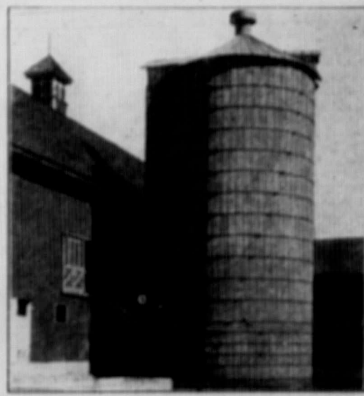
Concrete stave silo. There are a few of these in Manitoba and they have given good satisfaction. Better stock or better well concrete silos are really but fairly frost resistant and satisfactory.
