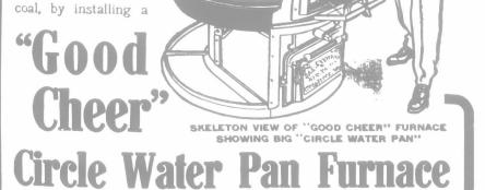
The evaporation from this big waterpan, which entirely surrounds the firepot and holds from 4 to 6 gallons, is sufficient to keep the warm air supplied to each and every room almost as humid as the outdoor air. That means genuine comfort without heating the house above  $68^{\circ}$  — and in consequence a substantial saving in coal.
