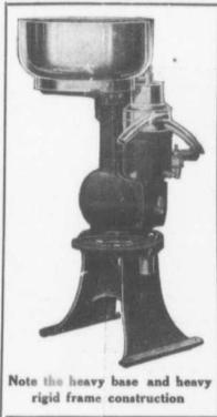
Note the heavy base and heavy rigid frame construction
