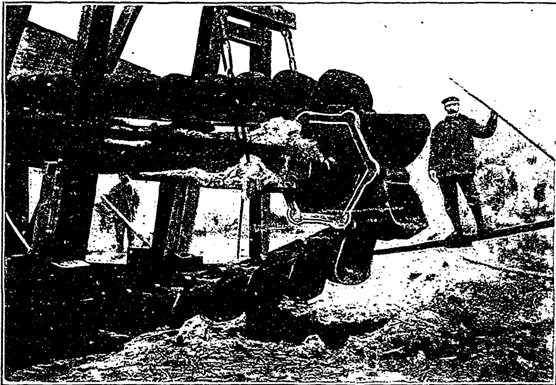
Buckets of the Robinson Gold Mining Dredge.
