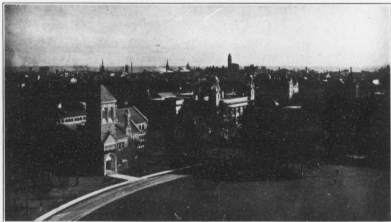
Bird's Eye View of University Buildings
