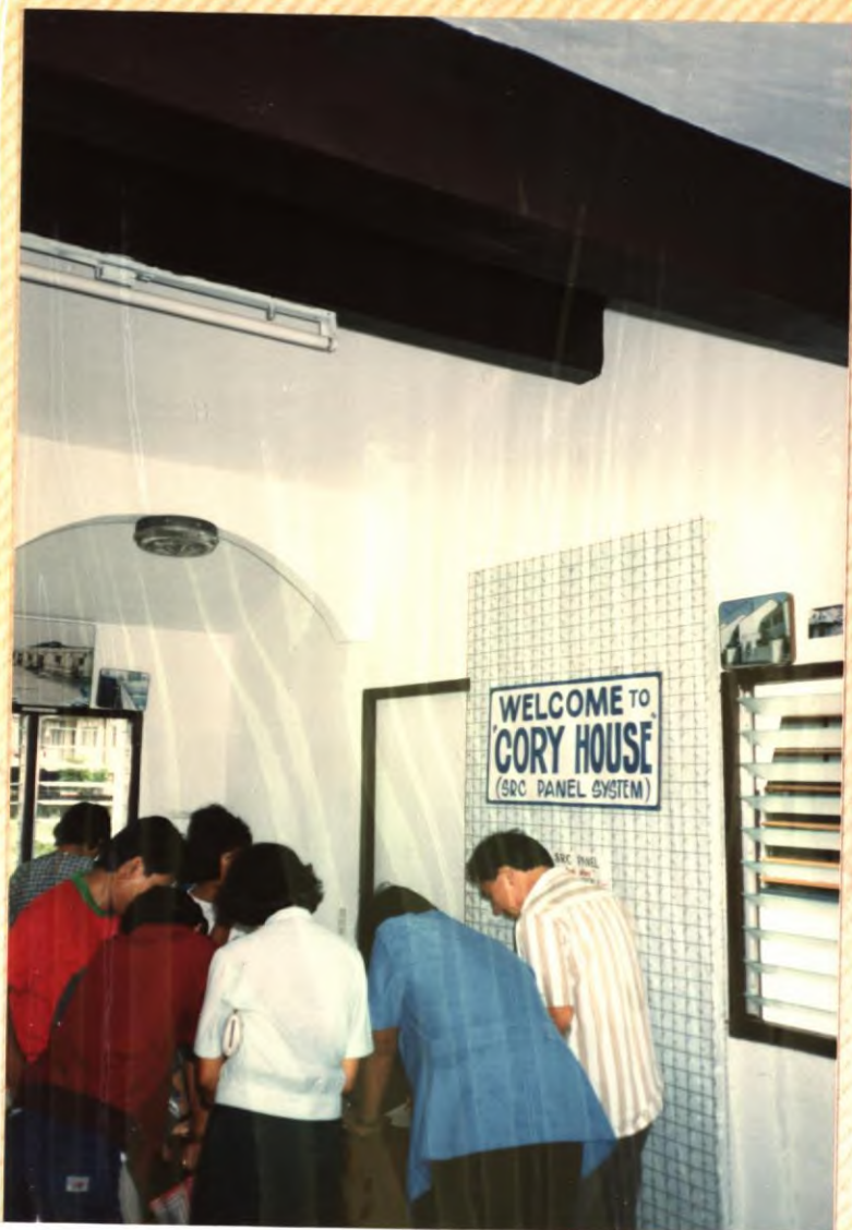
No. 38. Interior of Cory House showing SRC panel core before plaster is applied. People in picture are signing applications to purchase.
