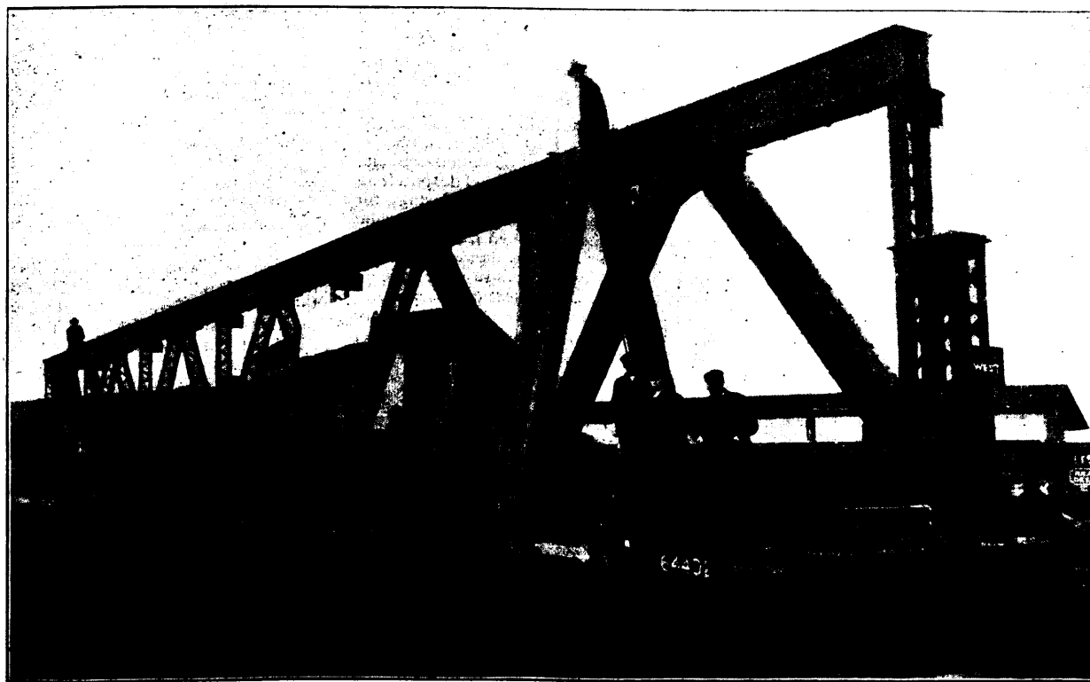
THE LARGEST BRIDGE TRUSS THAT HAS BEEN.
