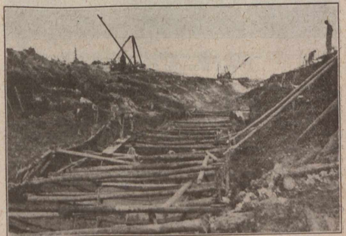
FIG. 6—SHEETING THROUGH SLIDE
