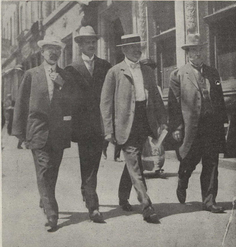
THE MEN BEHIND RIO.
