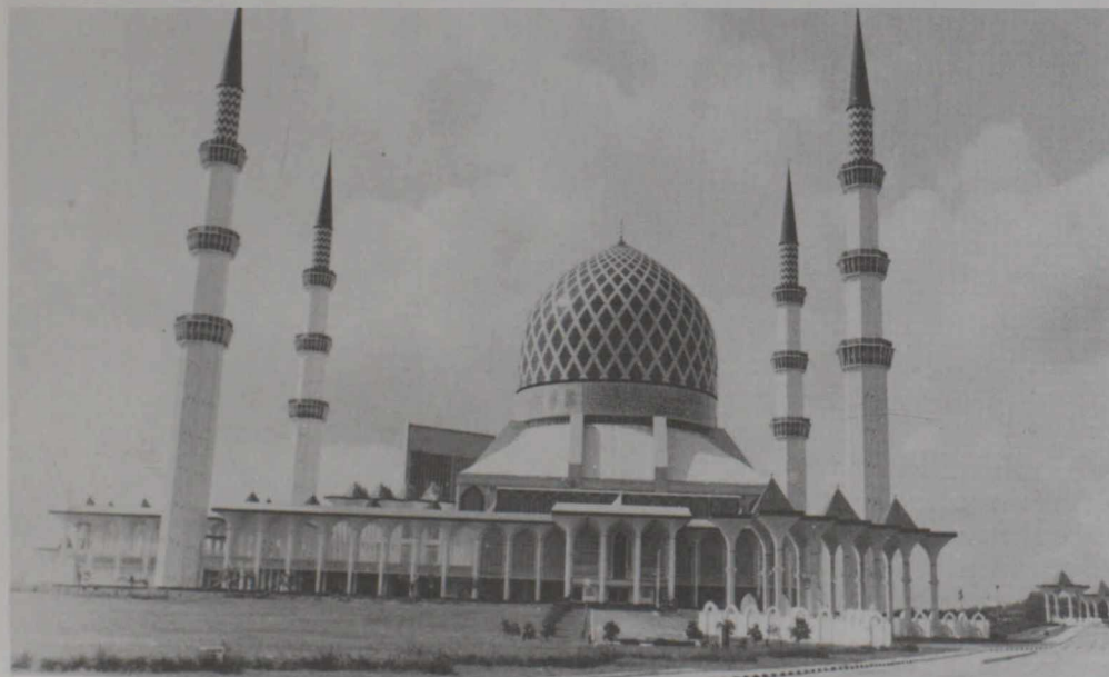
The attractive dome on the new Shah Alam Mosque was built using Canadian Triodetic technology.
