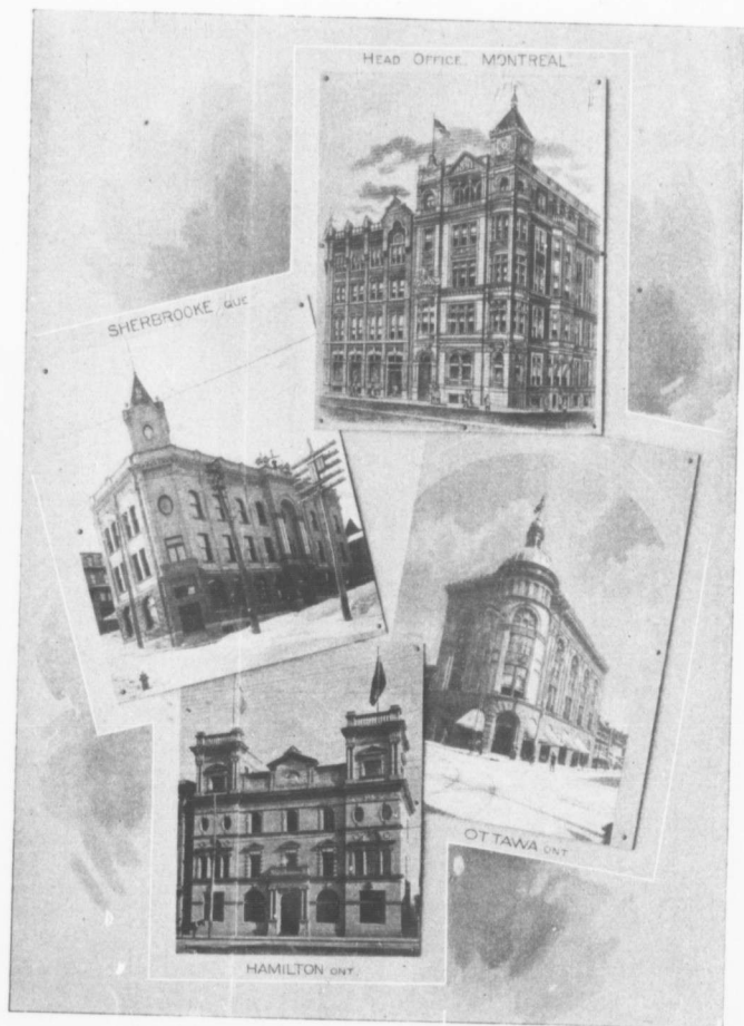
BUILDINGS OF THE SUN LIFE ASSURANCE COMPANY OF CANADA.
