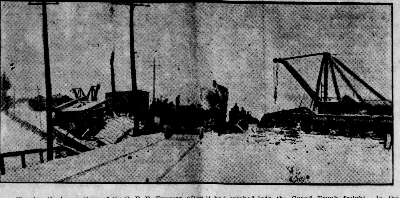
Showing the locomotives of the C. P. R. Express, after it had crashed into the bridge, and the wreckage of the train. The bridge was a close call for his life. The C. P. R. locomotive was not seriously damaged, losing only the smokestack, headlight, pilot, and a few minor parts.
