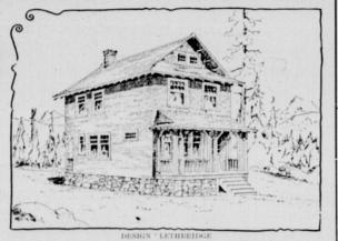
THIS ATTRACTIVE LITTLE HOUSE IS SHIPPED COMPLETE READY FOR ERECTION. ALL PARTS ARE MARKED CORRESPONDING WITH BLUE PRINTS, AND TALLY SHEETS SENT WITH SHIPMENT. ANY ORDINARY CARPENTER CAN ERECT IT.
