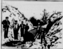
Here you see the Pedlar Culvert doing its work of drainage twenty-five minutes after being put in place. It would have taken three times as long and cost three times as much to have installed any other type of culvert. Yet this Pedlar Culvert will last far longer and give no further trouble of any kind.
