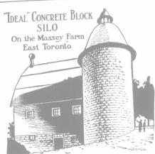
Erected at Dentonia Park Farm for Mrs. E. D. Massey. 34 feet high-15 feet diameter-capacity 180 tons. Built of "Ideal" Blocks.
