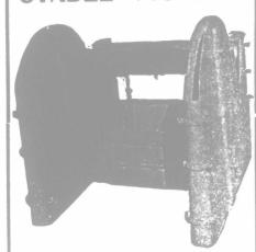
Adjustable mould for forming concrete mangers, stalls and water-troughs for cattle and horses. Pat. Oct. 24, 1909. For pamphlets, instructions to operate, and for prices, apply to
