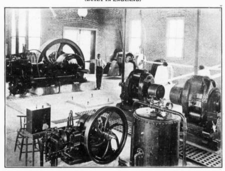
Interior view of Chatham, Ont., municipal street lighting station showing one engine (100 H.P.) countershaft, two of the series are machines, also independent petrol-engine-air-compressor and air container. At the opposite end of the room is another 100 H.P. suction gas engine. By actual test the fuel cost for 130 arc lamps was reduced from \$6.50 per day to \$1.00 per day.
