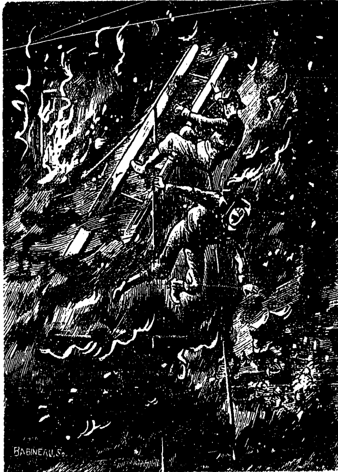
Two of our gallant firemen, T. H. Hogan and Wm. Stewart, of No. 3 station, jumping from a ladder in consequence of the fall of Kirkpatrick's cooerage, corner of Prince and Ottawa streets falling in on Thursday morning. They had a miraculous escape from death only having received a few injuries.
