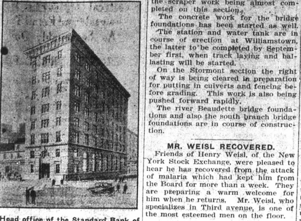
Head office of the Standard Bank of Canada, one of the newer buildings erected by various banking institutions in recent years in the Queen City.
