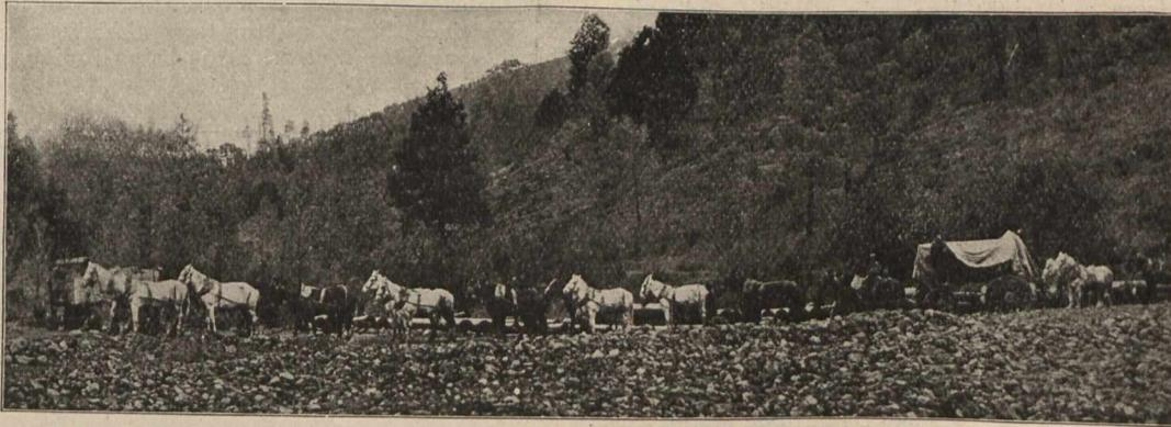
An 18-Horse Team Hauling the Lower Half of the Stator of an 750-k.w. Bullock Alternator Over 50 Miles of Mountain Road from the nearest Railroad Station to the Plant of the North Mountain Power Company.
