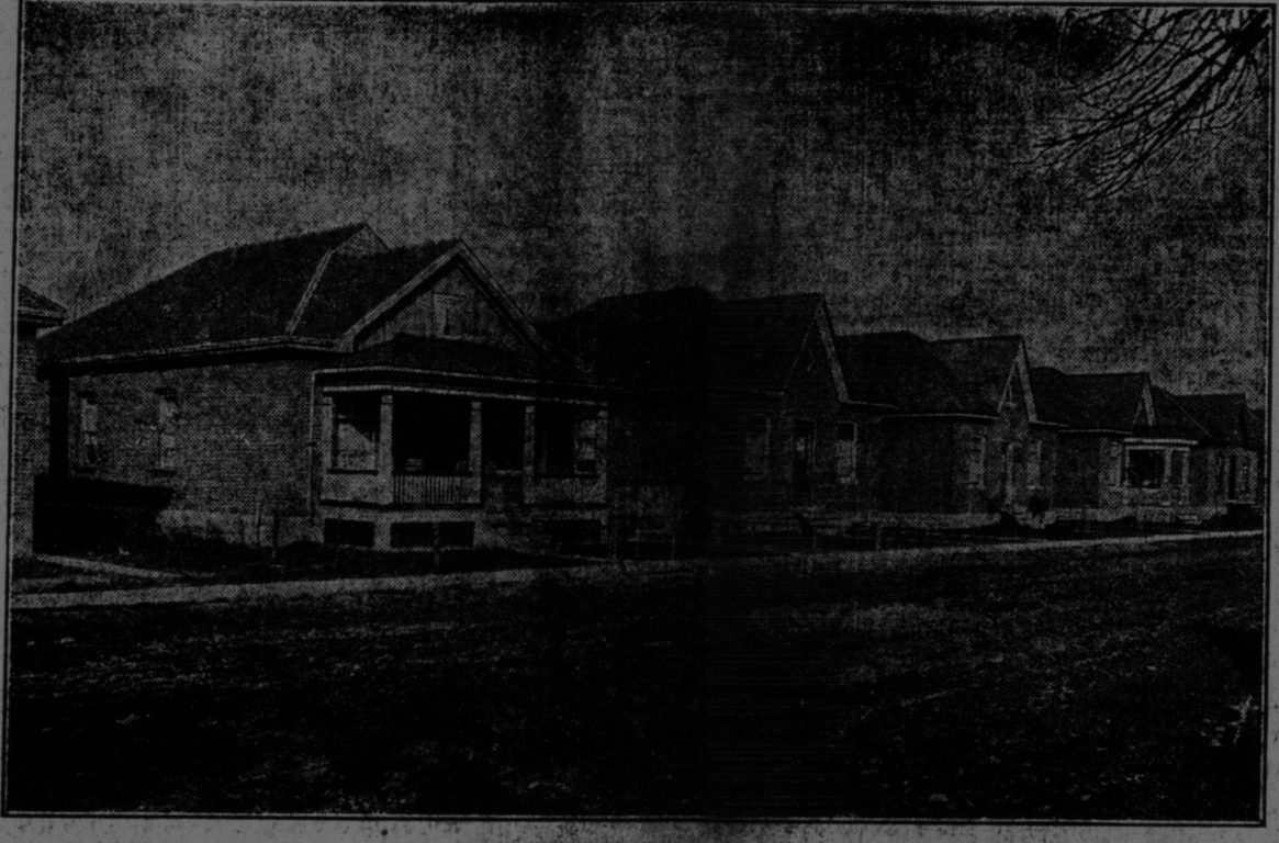
It has been said that cottages could not be built at St. John so fast as ten or twelve dollars a month. The two cottages in the middle of this picture were built to rent at that figure, and it will be observed that they are constructed of brick. Each of them contains six rooms. The picture is of a street in Brantford, Ontario, where practically all the working people live in separate cottages. They never see the habit of living in flats. On Monday the Times will show some Brantford cottages of a better class which rent at $12.50 a month.
