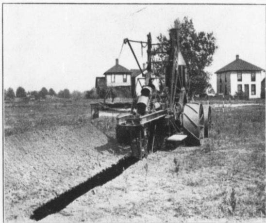
DITCHING MACHINE AT WORK.
