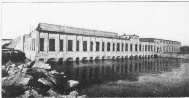
WINNIPEG RIVER—PINAWA CHANNEL STREET RAILWAY COMPANY'S POWER HOUSE, SHOWING TAILRACE
