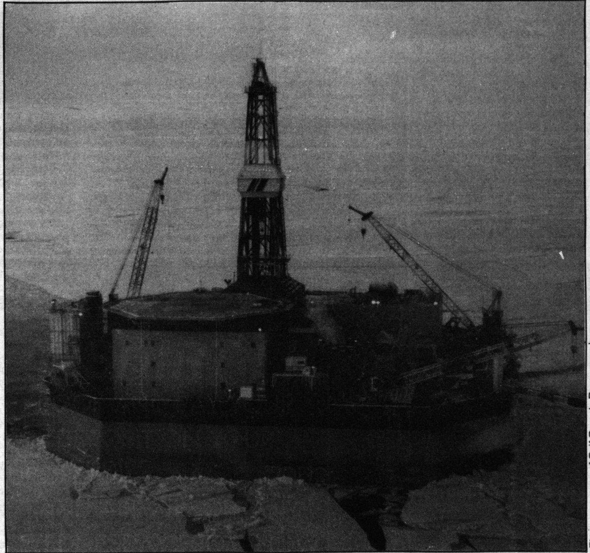
The need for ice protection is evident in this photo of Gulf's Molikpaq drilling rig.
