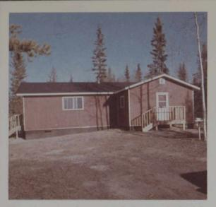
The red house shown here was built by Beavers at Peerless Lake in Northern Alberta, with help from local people, for under \$13,000 in materials. It is framed in 2 x 6s. With R20 insulation and a wood-burning heater, it is snug at  $40^{\circ}$ F below.
