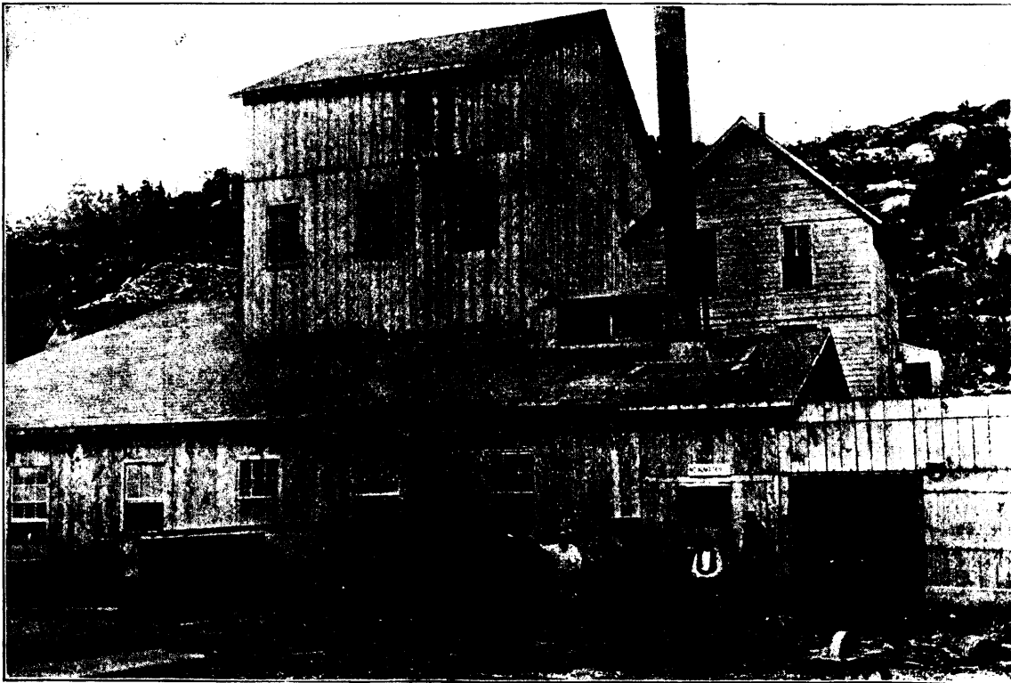
10 Stamp Mill at Sultana Mine.
