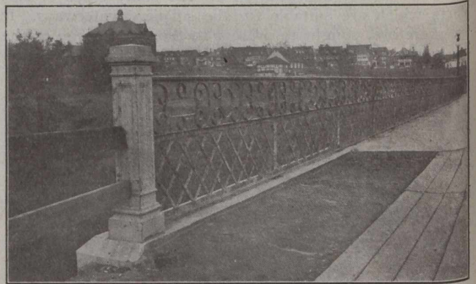
Steel Lattice Handrail.
