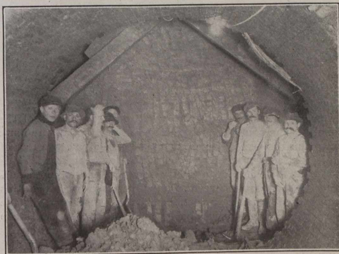
Fig. 7.—A Portion of the Work Required Very Little Sheeting Owing to the Favorable Nature of the Clay.
