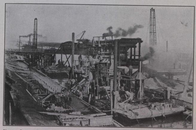
Fig. 1.—Concrete Handling Plant at Work on Don Diversion Channel Walls, Toronto Harbor Commission.
