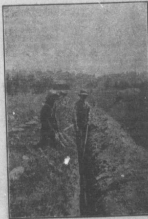
Mr. Dawson Grading a Ditch Bottom.
