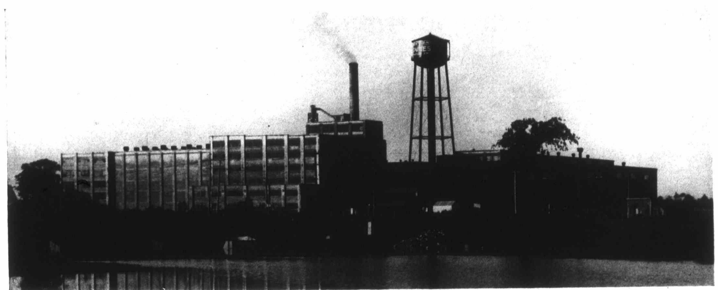
Huge New Plant at Farnham for Manufacture of Linoleum. Just a little over three years ago, in October, 1931, this large factory with floor area of 262,084 sq. ft. started operations at Farnham, Que. It is the Canadian headquarters of Barry and Staines Linoleum (Canada) Limited and gives employment to some 120 hands.
