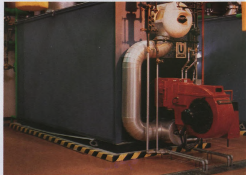
The high-efficiency watertube Unilux boiler is available in capacities of up to 1 200 hp.
