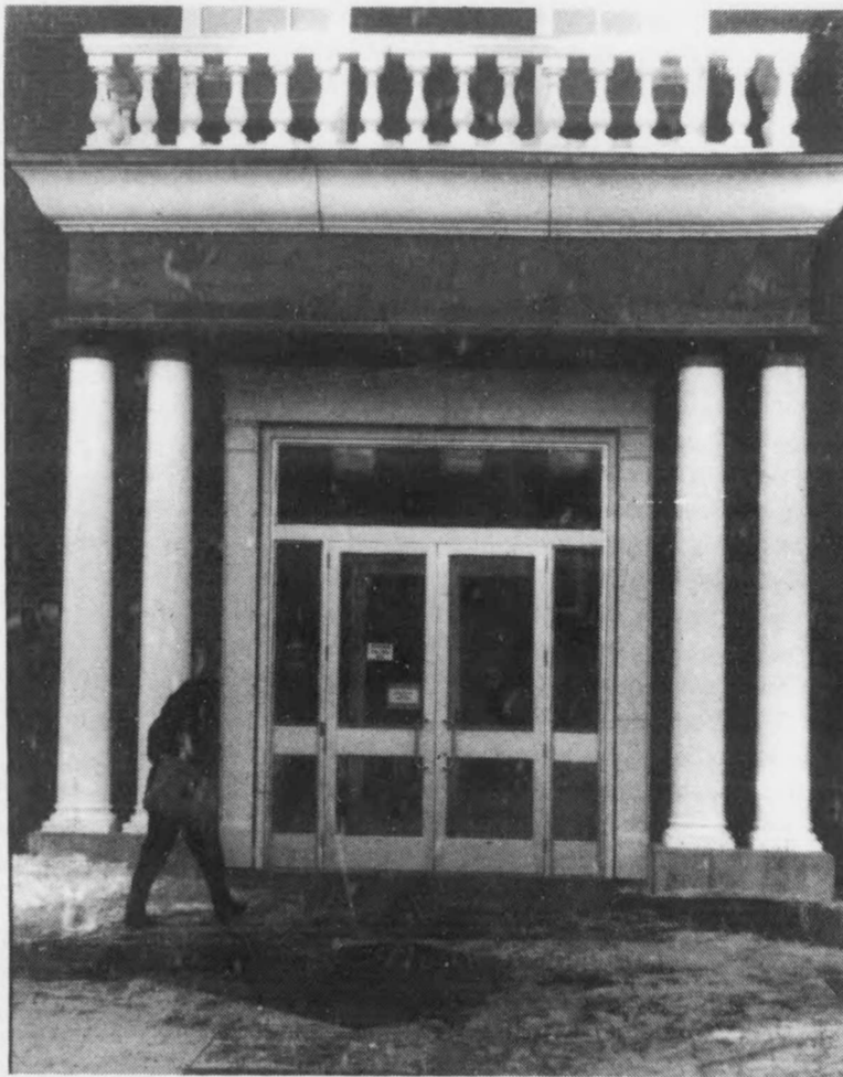
Entering the front doors of the now completed Sir James Dunn Hall, the name remains to be affixed. Photo by Marc Landry
