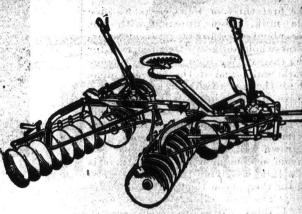
suitable for horse or engine power. By grouping four, six or more harrows together you can do double action work on a large scale. Write Dept. T. for further information-
